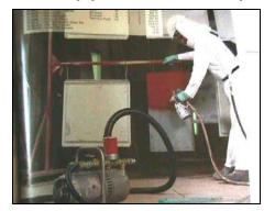
SARs, like SCBAs, provide the highest level of respiratory protection. An SAR includes a full face piece connected to an air source that is away from the contaminated area.
